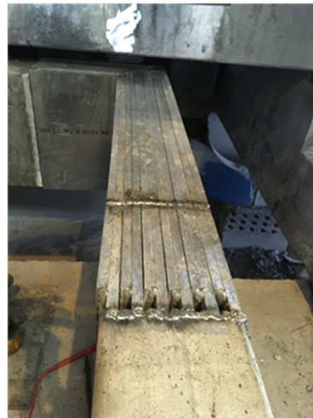
Figure 8. Bus bar after its welding repair (located under the potshell).
