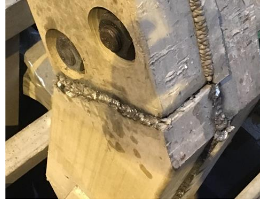
Figure 10. Anode Riser C located in the middle of the pot.
